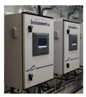
Excellent performance for multigas measurements in dry sampling, including HCL, HF, NO, NO<sub>2</sub>, N<sub>2</sub>O, SO<sub>2</sub>, CO<sub>2</sub>, TOC, CH<sub>2</sub>, CO, O<sub>2</sub>.
