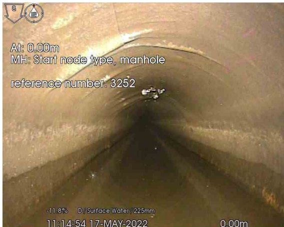
3252_0-00m_111454.jpg, 00:00:00, 0.00 m Start node, manhole, reference: 3252
