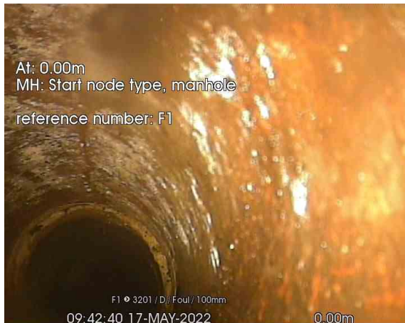
F1_0-00m_094240.jpg, 00:00:01, 0.00 m Start node, manhole, reference: F1
