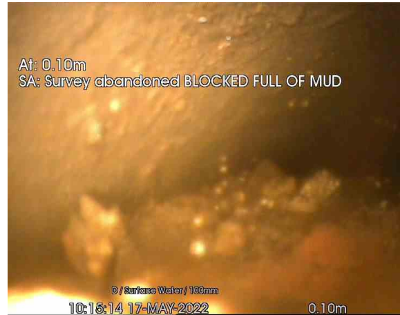
GY2_0-10m_101514.jpg, 00:00:42, 0.10 m Survey abandoned, BLOCKED FULL OF MUD
